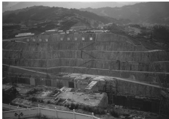
Fig. 11. View of excavated shiplock slope
