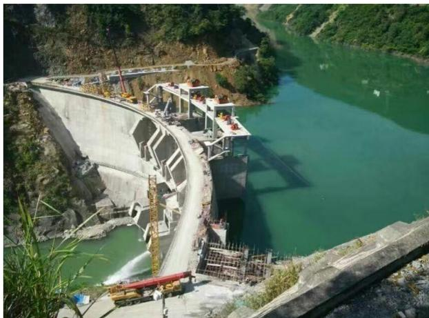
Figure 2: Baijia RFC arch dam completed in 2015
