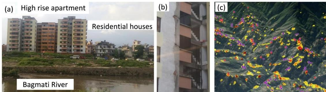
Figure 6: Overview of high rise apartment and low rise residential building in Buddanagar, Kathmandu, (b) severe cracks on high rise apartment, and (c) Ridge-top damage interpreted from satellite image decorrelation before and after the main shock (ARIA/JPL-Caltech)
